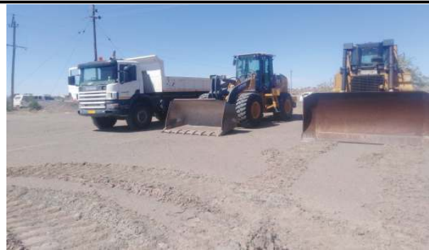
Photo No. 2: Plant mobilization
