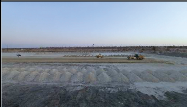
Photo No. 8: Process roll and compact 150mm platform layer.
