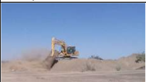
Photo No. 8: Ponds Excavation & Stock piling all insitu material.
