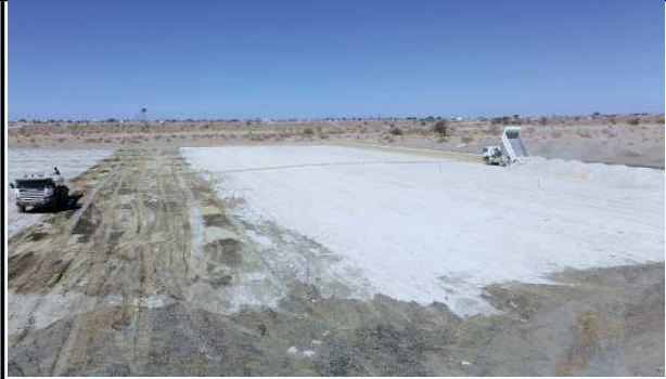
Photo No. 2: Wetting and processing of 150mm Blanket layer
