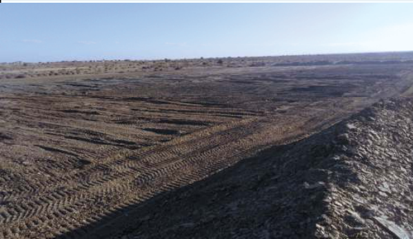
Photo No. 5: Levelling of pond Platform layers.
