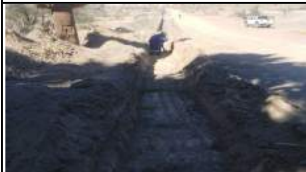
Photo No. 5: Trimming and preparing trench for bedding
