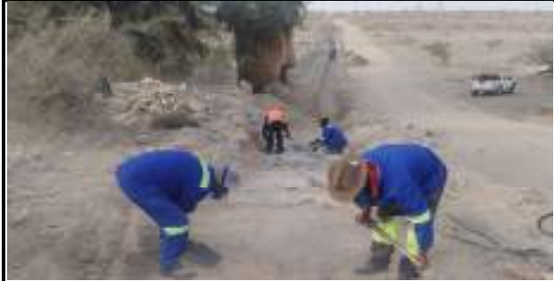
Photo No. 3: Exposing hard rock for Excavation
