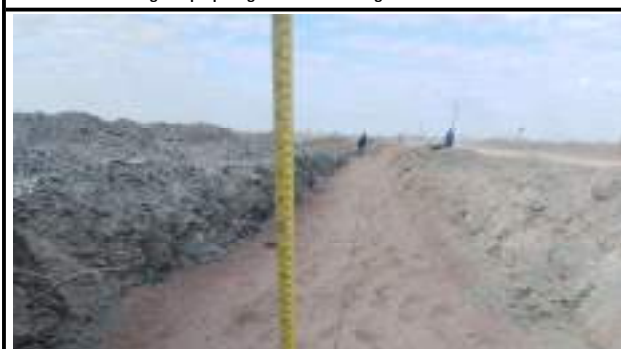
Photo No. 7: Trench bedding
