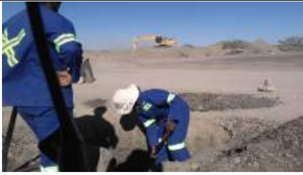
Photo No. 1: Exposing all existing services
