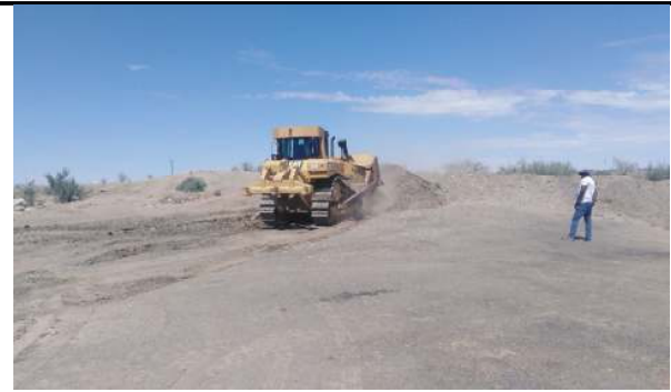
Photo No. 6: Site clearance
