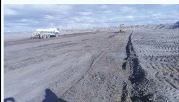
Photo No. 6: Water and preparation of pond bed.
