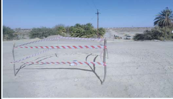
Photo No. 2: Leveling and demarcating of feeder pipeline
