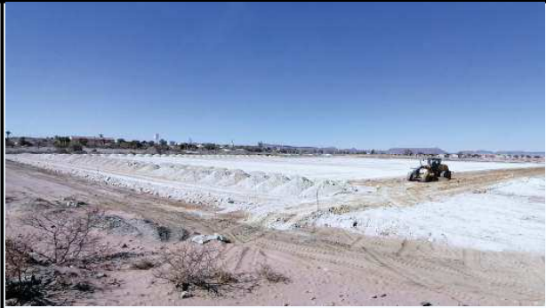
Photo No. 4: Preparation of embankments floors.
