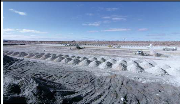
Photo No. 7: Processing of blanket layer and hauling of Embankments material
