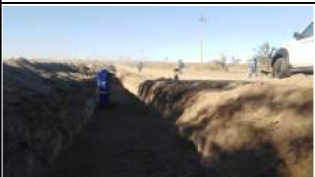
Photo No. 6: Leveling of trench
