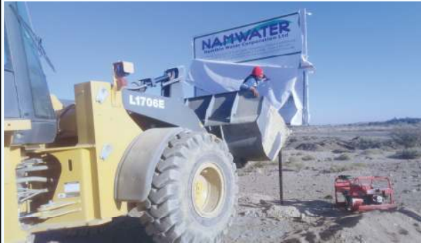
Photo No. 1: Erecting of Project Nameboard
