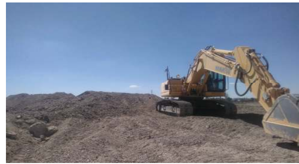
Photo No. 8: Ponds Excavation to platform level.
