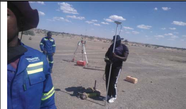
Photo No. 5: Setting out
