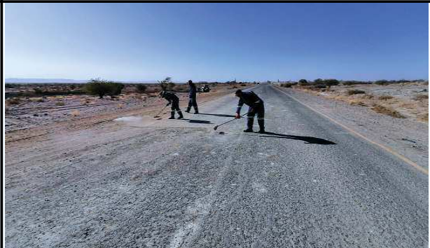
Photo No. 6: clearing of section of hauling at road crossing section.
