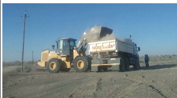
Photo No. 7: Site clearance
