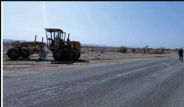
Photo No. 5: Maintenance of hauling route from borrow pit.
