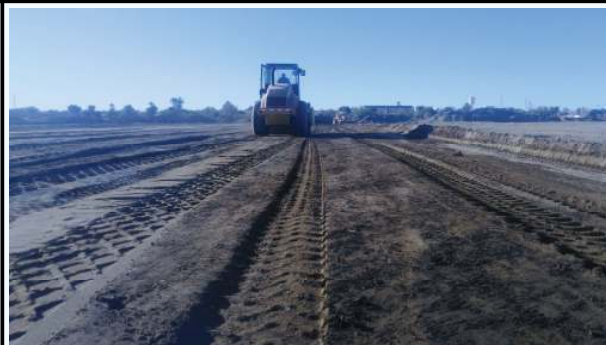
Photo No. 8: Roll and compact platform layers
