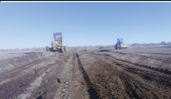
Photo No. 7: Procecing of platform layers.
